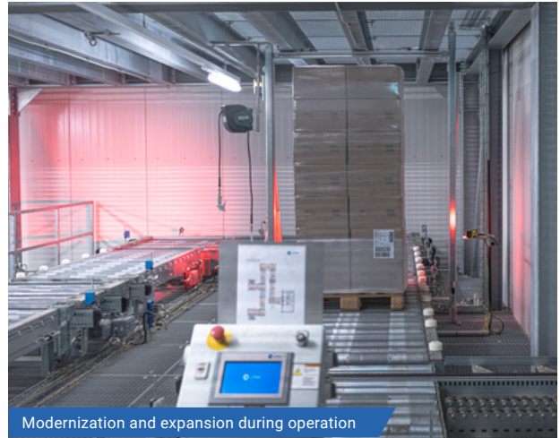
Modernization and expansion during operation
