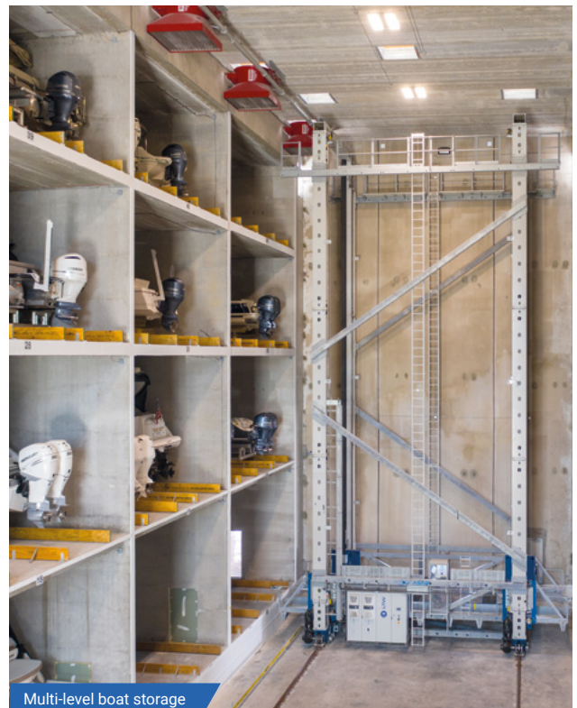
Multi-level boat storage
